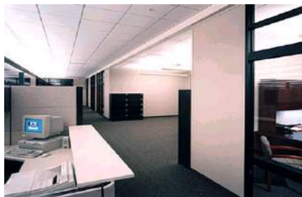
Movable partitions cost more than studwork, the extra cost buying the lifecycle option to rearrange the office layout economically and with minimum disruption.
