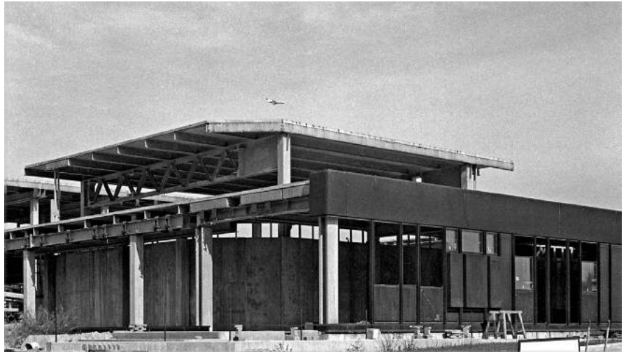
A classic case of over-investment in flexibility: the Free University of Berlin by Candilis Josic Woods, built in 1967-74 (photo 1970), made the common mistake of confusing the objective of flexibility in use with the provision of elaborate and expensive hardware for physical change.
